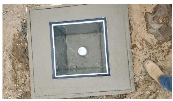
Photo 13. 2'x2'x2' traffic rated vault set in concrete (vault lid not in view).
