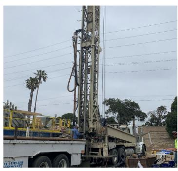
Photo 2. Mud rotary drilling setup. Pilot hole drilling in progress.
