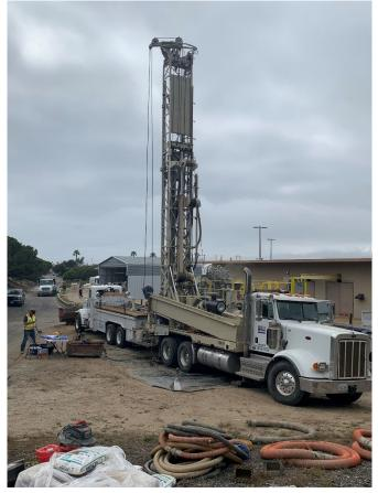
Photo 3. Mud rotary drilling setup. Pilot hole drilling in progress. Note geologist logging table on left.
