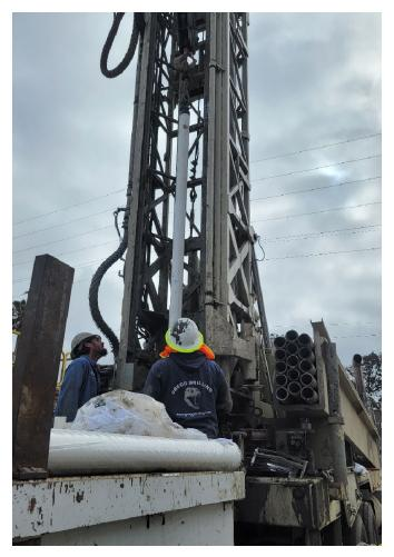
Photo 9. Installing PVC well casing.
