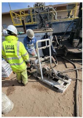
Photo 11. Pumping bentonite chips into borehole to seal between aquifers.
