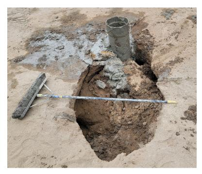
Photo 4. View of sinkhole after safely removing drill rig. Note secondary conductor casing installed to stabilize drill hole.
