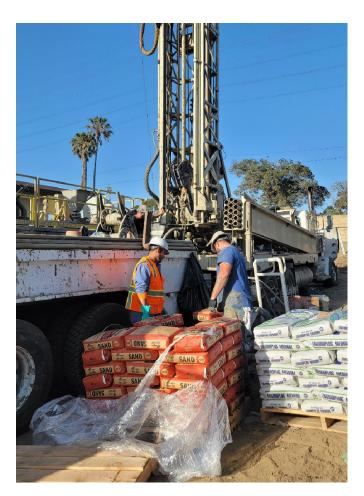
Photo 10. Preparing to install sand filter pack around well screen.
