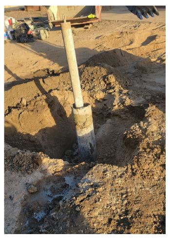
Photo 12. Excavating around well for vault installation.
