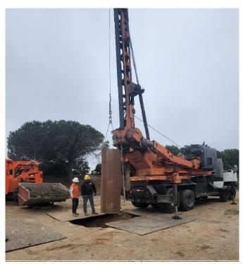
Photo 1. Installation of conductor casing
