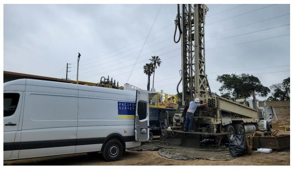
Photo 8. Performing geophysical survey of borehole to inform well design.
