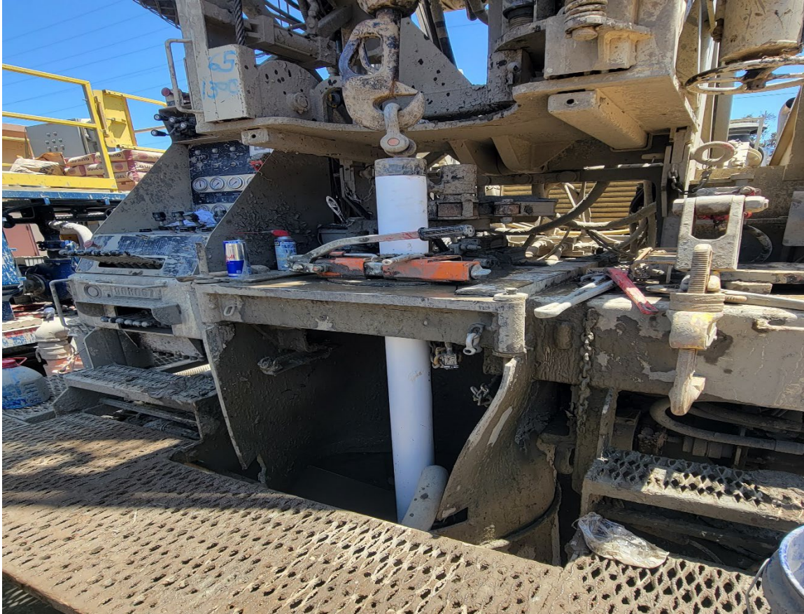
Photo 9. Well Casing Installation
