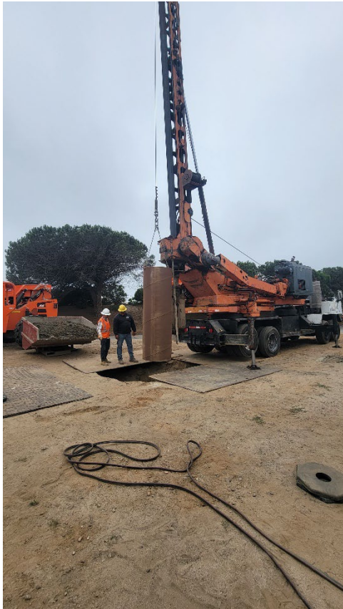
Photo 1. Bucket Auger Rig Setup to Install Conductor Casing.
