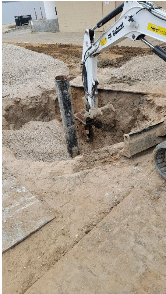
Photo 7. Backfilling Sinkhole
