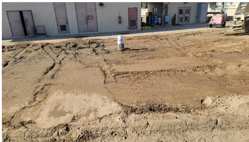
Photo 7. Backfilling Sinkhole
