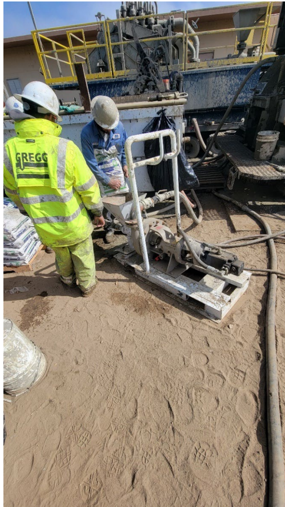
Photo 10. Setup to Install Filter Pack
