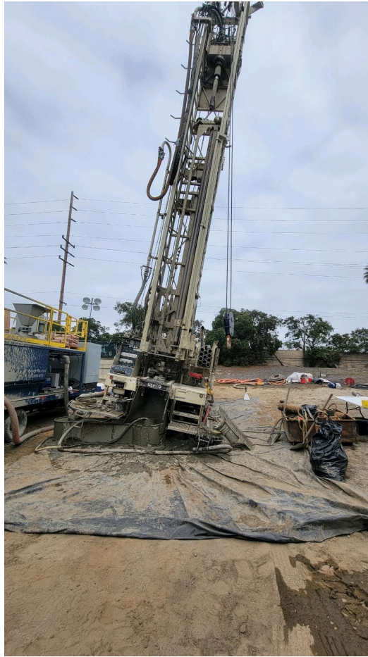
Photo 5. Leaning Rig due to sink hole.
