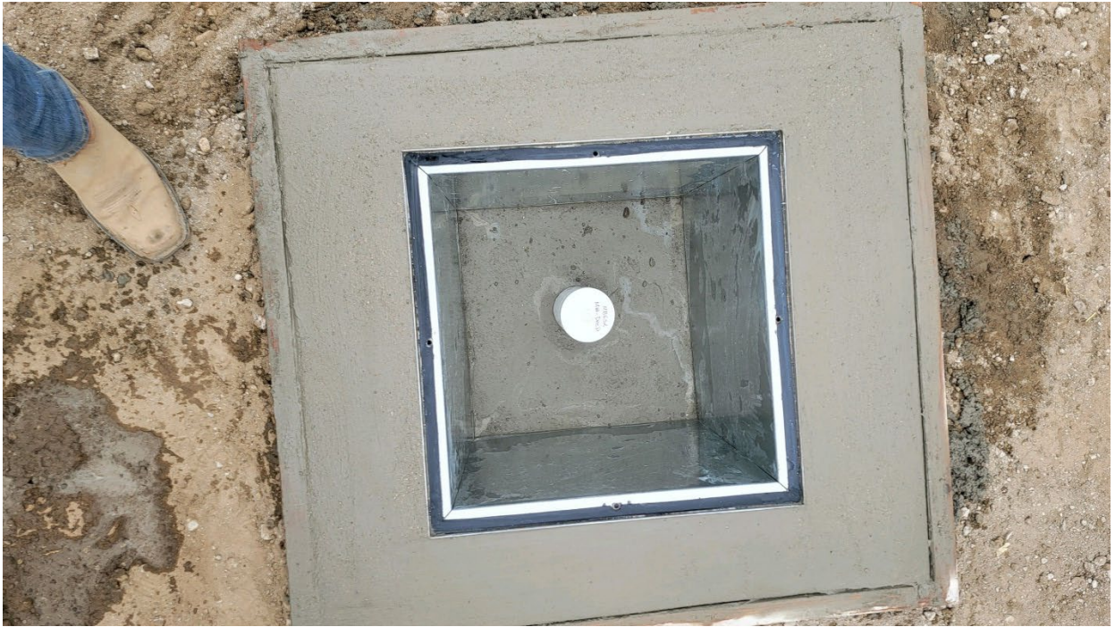
Photo 11. Setting 2'x2' Well Vault in Concrete
